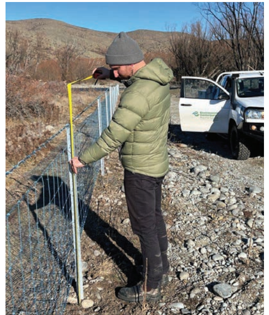
Checking the construction height of the wallaby exclusion fence at 1.3 metres.
